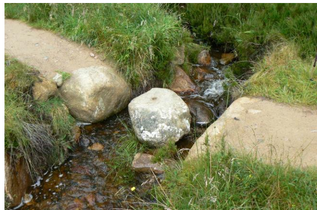
30 OPEN DRAIN CROSSING CONSTRUCTED USING LARGE BOULDERS.
