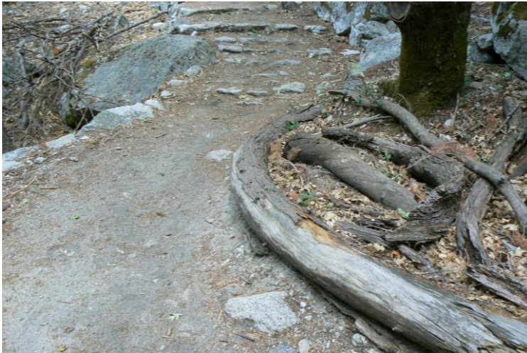
92 USING THE NATURAL SHAPE OF THE LOG GIVES VERY EFFECTIVE PATH DEFINITION
