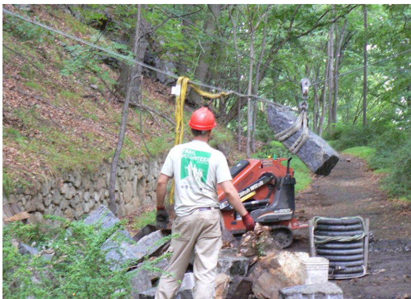
17 MOVING MATERIALS ONTO THE WORK SITE CAN BE COSTLY AND SLOW IN REMOTE OR DIFFICULT AREAS. A trail builder moving rock with a cable system on the Appalachian Trail at Bear Mountain, N.Y.
