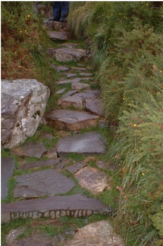
48 STONE PITCHED TRAIL - Torc Mountain Path, Killarney National Park, using imported rock.
