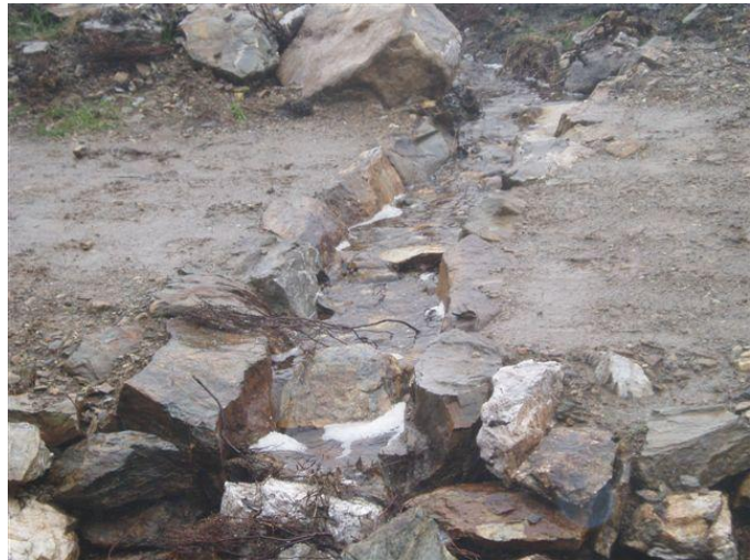
29 STONE CROSS DRAIN (Photo Shay Walsh)
