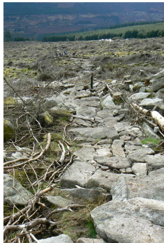
49 STONE STAIRCASE This trail was built with local material arranged in such a way as to form a very durable walking surface. (Curtlestown Forest, Glencree, Co. Wicklow)
