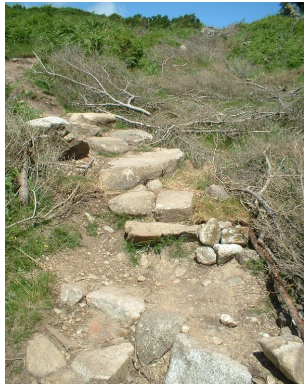
89 BRASH used to keep walkers on the steps and off a re-vegetation zone. (Photo Shay Walsh)
