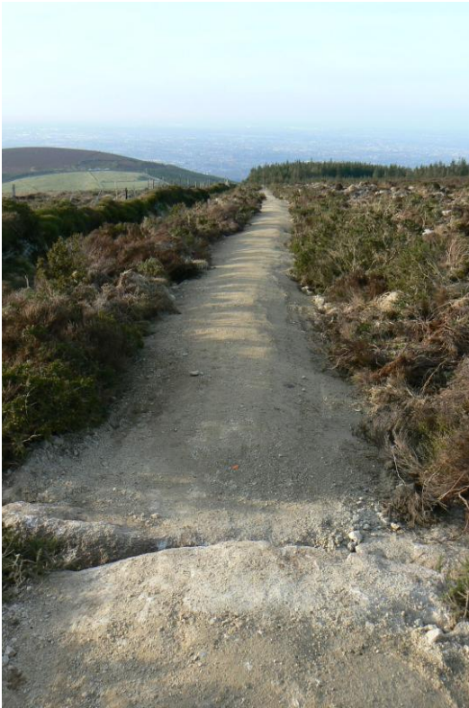
45 COMPLETED REVERSAL TRAIL - note the landscaped edges to the trail and the stone waterbar in the foreground.
